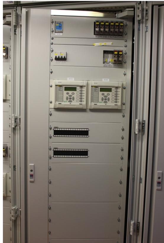
Figure 12: 50Hertz standardized protection panel for transformer protection
