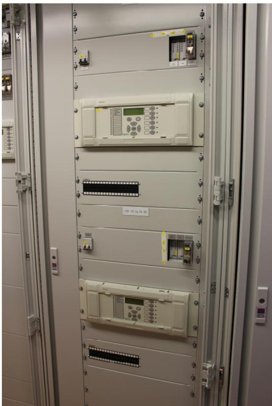
**Figure 13: 50Hertz standardized protection panel for line differential protection**
