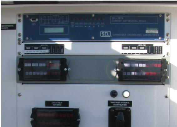
**Figure 8: Example of a EKPC protection panel with standardized test access points**
