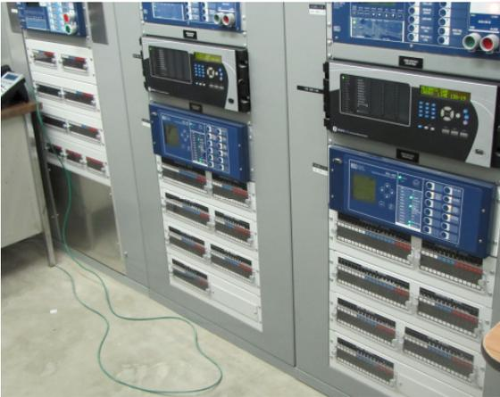
**Figure 10: Example of TNMP test block installations**
