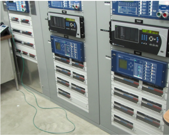
Figure 10: Example of TNMP test block installations
